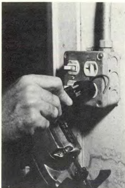
Adapter should be used to update old style electrical outlets. When shifted from outlet to outlet ground wire soon breaks.
