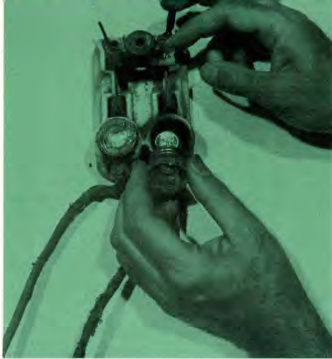
The "penny behind the fuze" syndrome. Known to be the cause of many catastrophic fires. Deteriorated wire insulation will help bring on disaster.
