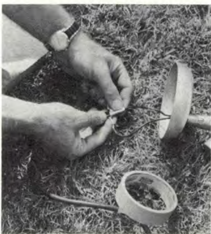
Never, but never, use masking tape on electrical connections but that's not all . . . although the next guy solders connection (use only rosin core solder) and electrical tape—he's still dangerous. This fixture is designed to mount on a properly wired box, not attach to a cord!
