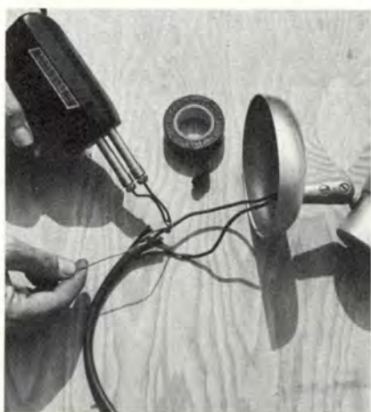
Never, but never, use masking tape on electrical connections but that's not all . . . although the next guy solders connection (use only rosin core solder) and electrical tape—he's still dangerous. This fixture is designed to mount on a properly wired box, not attach to a cord!
