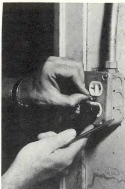
Ground wire should be attached to outlet box if house is wired with conduit. If conduit is not used, best have circuit rewired.
