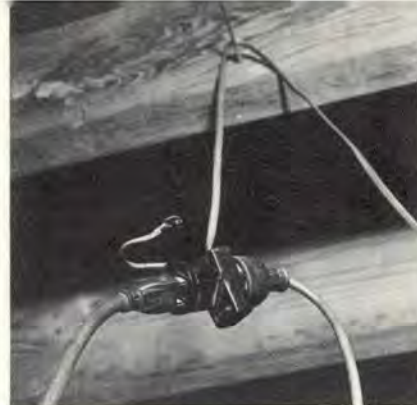
Typical "do it yourself" installation by a home handyman. The possibilities for fire are frightening.
